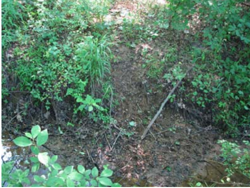
Figure 14: Erosion due to Animal Crossing
